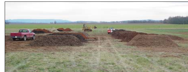
Installation of AL A&M field study site.
