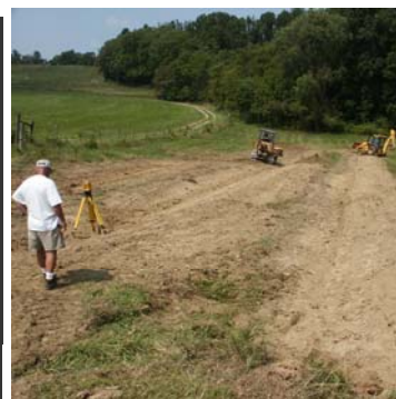
Waterway Construction August 2005
