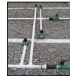
FIG 4 – Solenoid valves were used in combination with a misting controller to initiate 30 second irrigation cycles daily.
