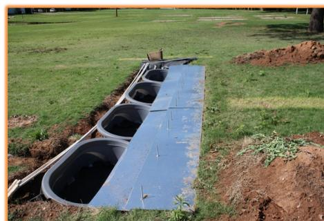
Photo 1. Metal plates and shingles conduct raw runoff into filter tubs
