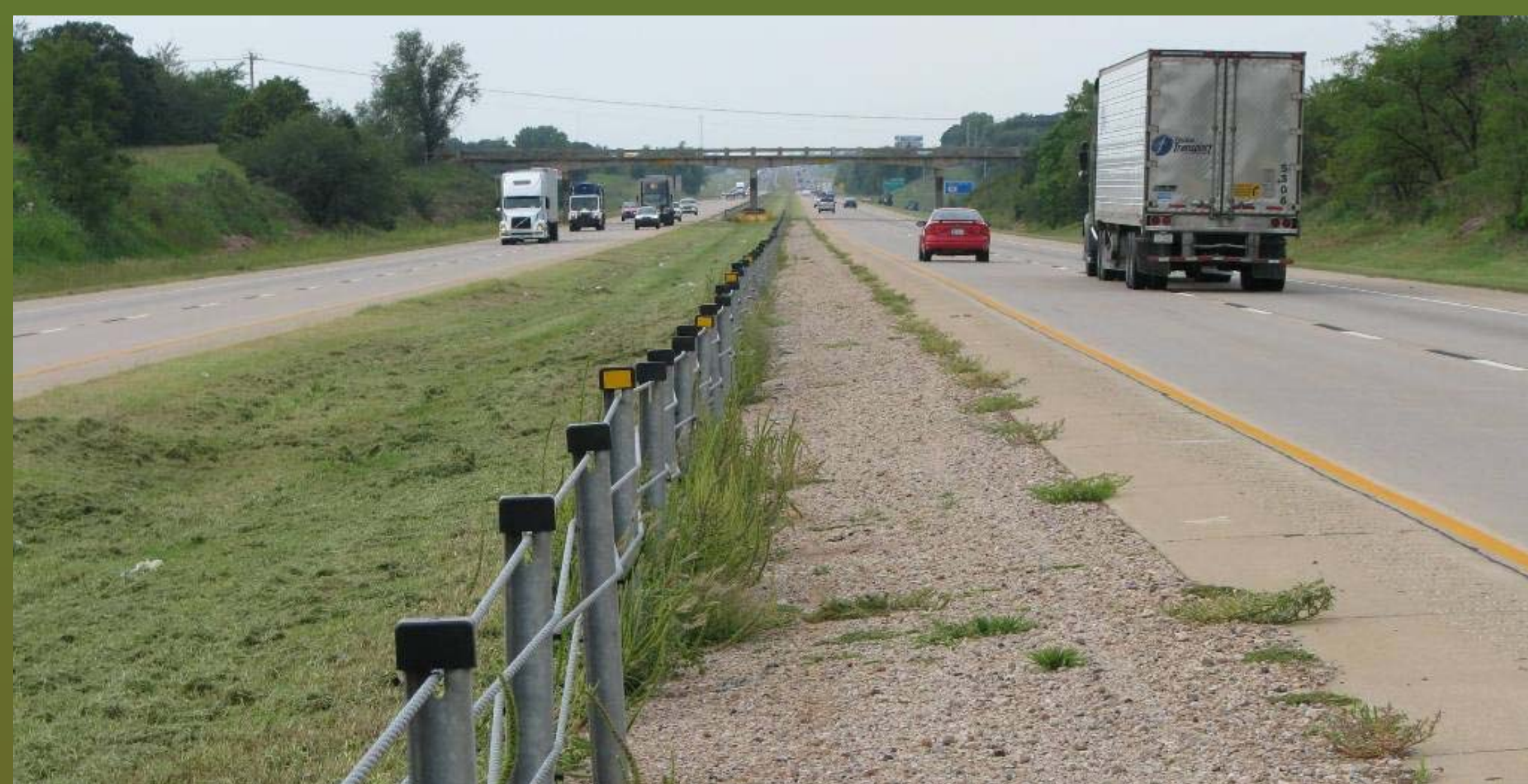
Figure 1. Roadside vegetation managers face many challenges including weed control and mowing requirements in roadside turf as well as weed invasion along cable cross-over protection barriers. Vegetation encroachment into the cracks and seams in concrete and asphalt pavement will eventually destroy the pavement over time if left unmanaged.
