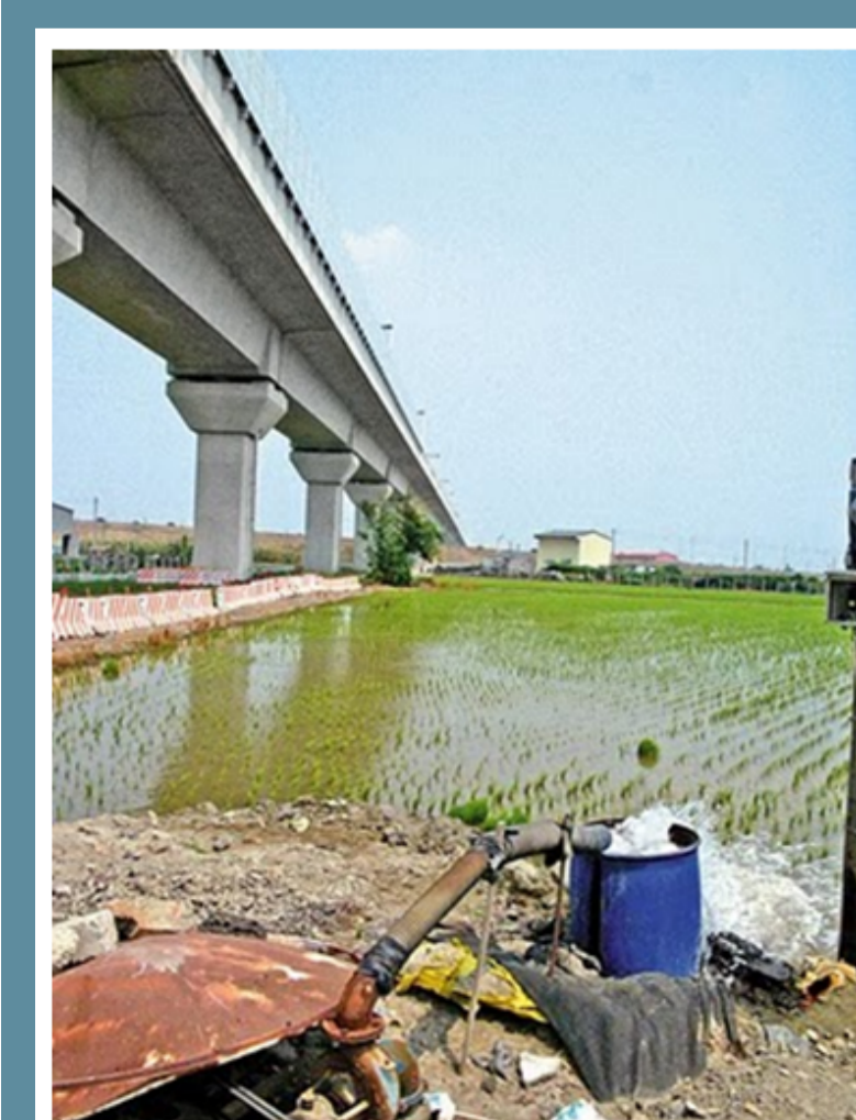
Figure 2. agriculture well and the hose with serious land subsidence
