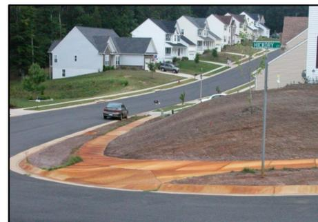
Active acid sulfate soils in Great Oaks development, Fredericksburg, VA. Sidewalks turned red from oxidation and hydrolysis of iron in seepage waters released by oxidation of iron sulfides in soil exposed by excavation; waters were partially neutralized by concrete.
