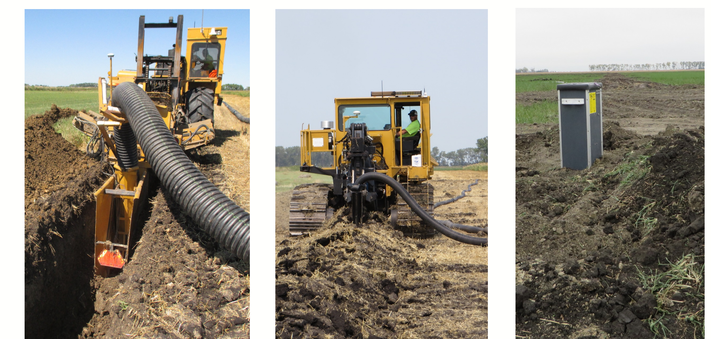
Figure 5. Trenching in 12 inch main line (left), plowing in 6 inch sub-main line (center), water control structure after installation (right).
