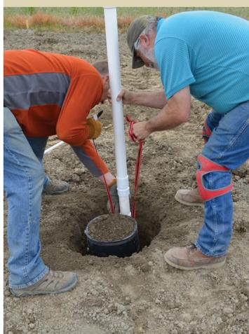
Installing drain gauge at Washington
