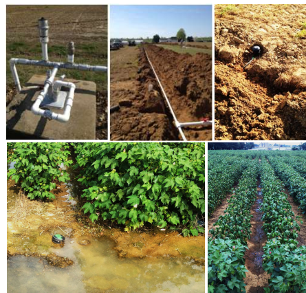
The sub-surface drip irrigation regimes system at WTREC designed and assembled by Tennessee Tractor LLC - Jackson John Deere Dealership
