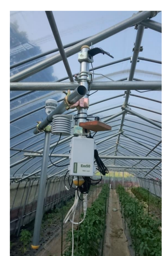
Environmental condition sensors
