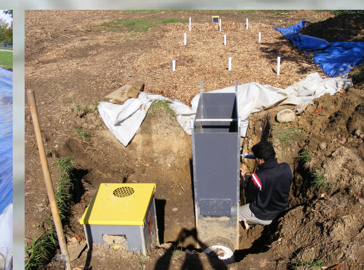
Another view of the agricultural tile bioreactor showing inlet structures located in front of bioreactor.
