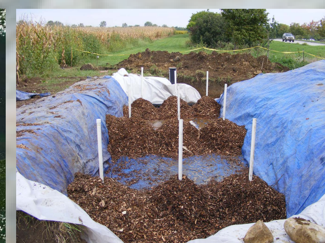
Installation of agricultural tile bioreactor at Waterman Farm, The Ohio State University Columbus Main Campus. Designed to remove both dissolved reactive phosphorus and dissolved nitrates.
