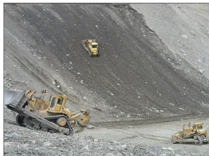
Figure 2: Reestablishing approximate original contour
