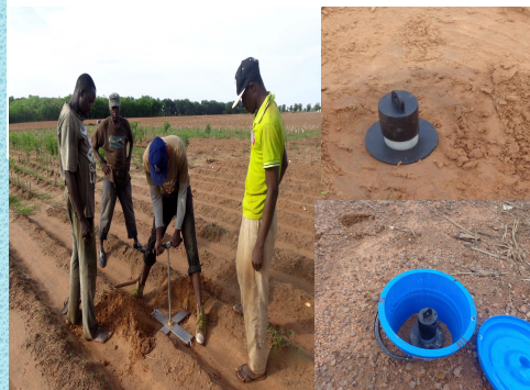
Figure 1. Access tube installation
