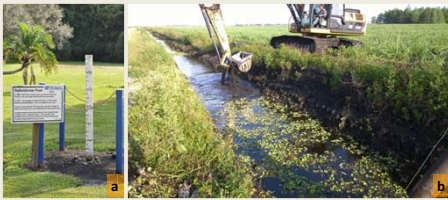
Fig 1. a) Soil Subsidence and b) aquatic vegetation in canals.
