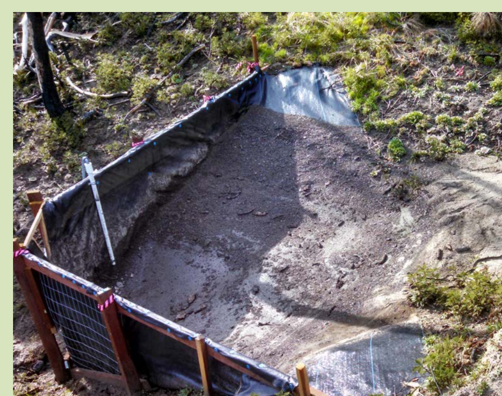
Fig. 3: Silt fence at outlet.
