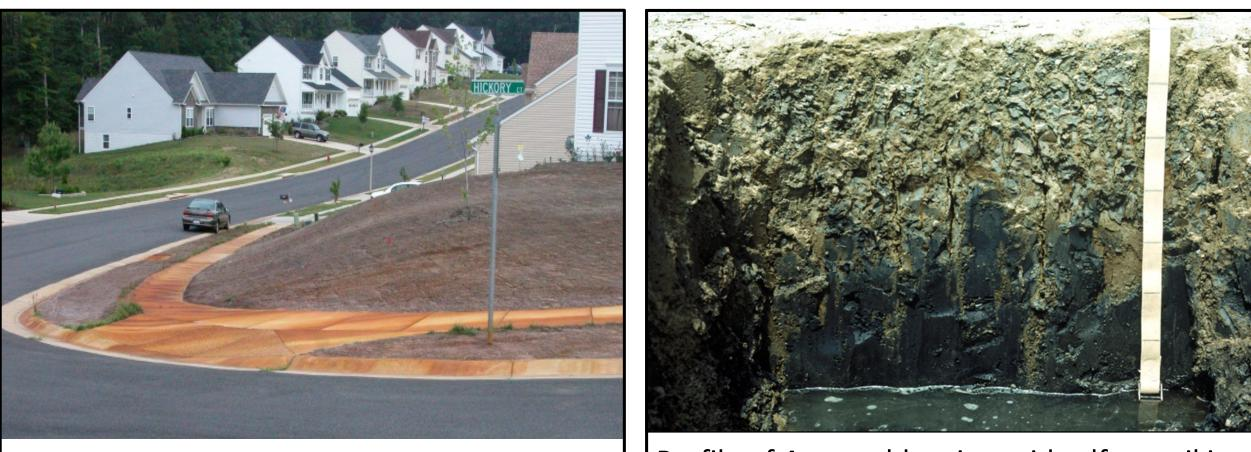
Active acid sulfate soils in Great Oaks development, Fredericksburg, VA. Sidewalks turned red from oxidation and hydrolysis of iron in seepage waters released by oxidation of iron sulfides in soil exposed by excavation; waters were partially neutralized by concrete.
