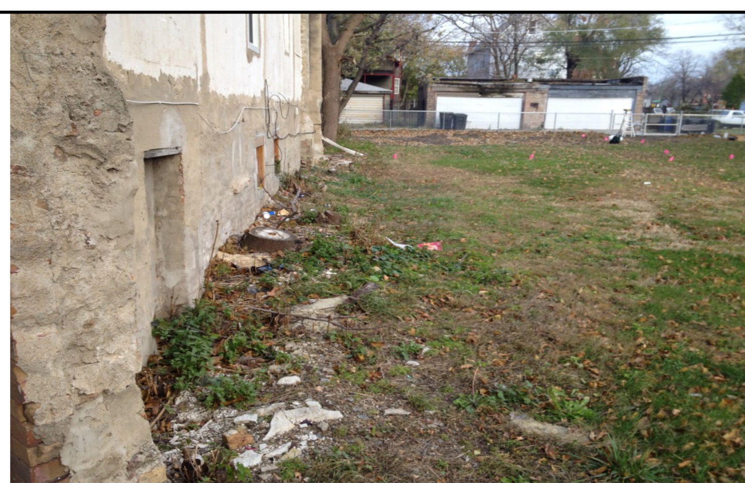
Figure 2a. Abandoned residential lot littered with demolition debris in Grand Crossing.
