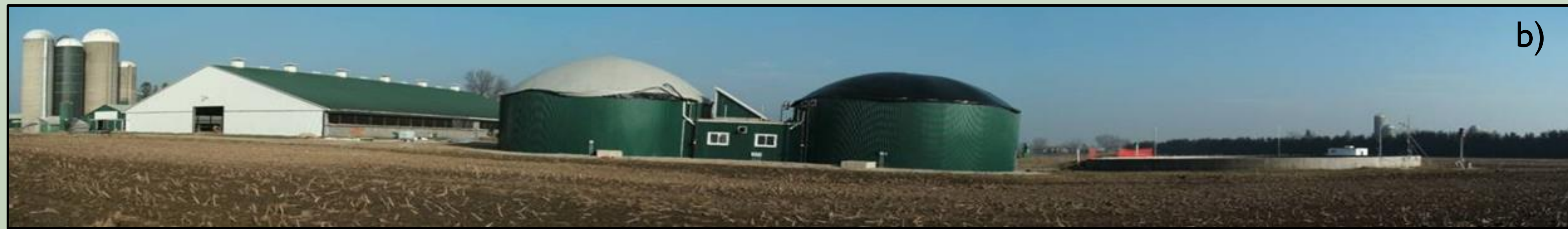
Figure 1 – a) Map of AD system components, with wind sectors contributing to each method. b) Photo of AD system in 2012. Left: barns and mixing tank. Centre: two-stage AD unit. Right: storage tank.
