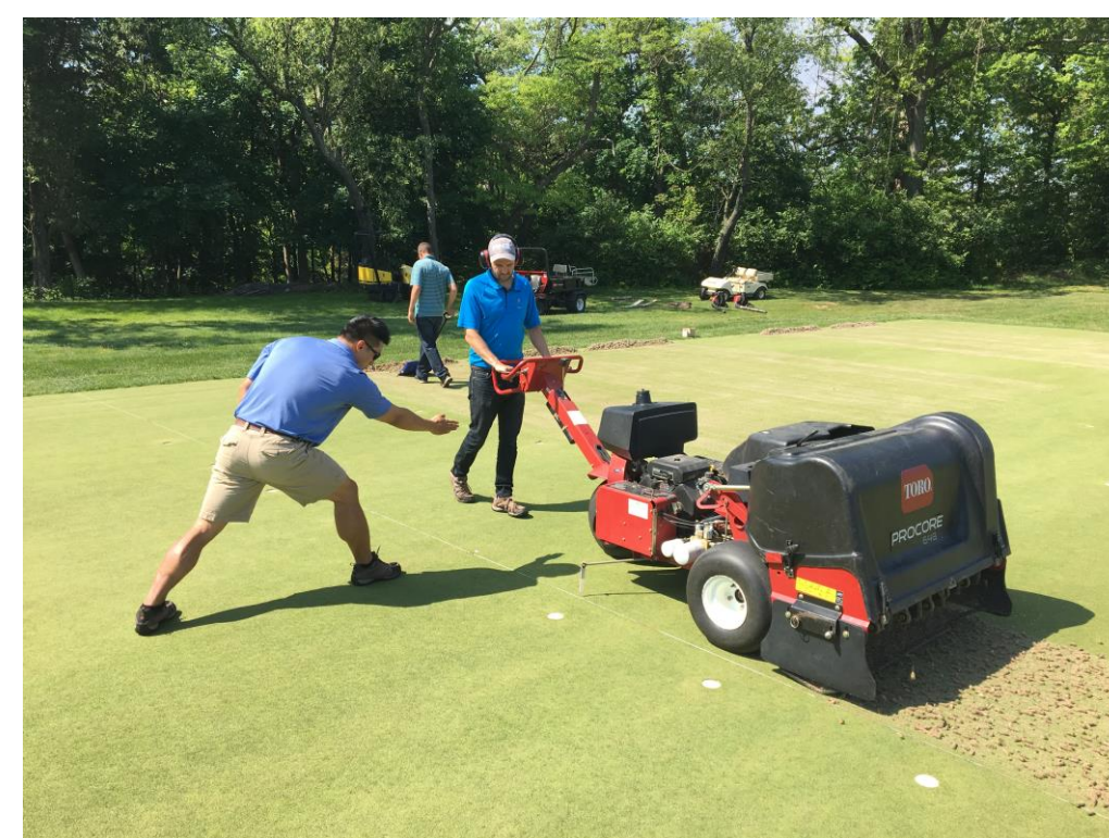
Core cultivation before backfill.
